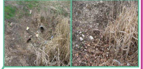
Outfall #5: Star Rd. and Heath Way south side of intersection
