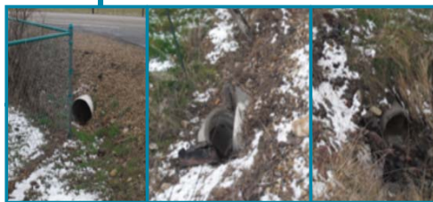
Outfall #6: Lewis Ln. and 12th Ave. Drain
