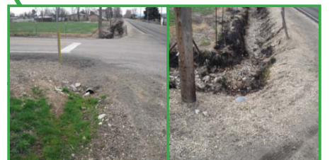
Outfall #10: Orchard Ave. and Pit Ln.
