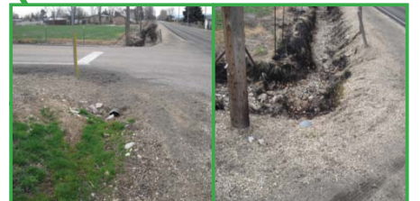
Outfall #10: Orchard Ave. and Pit Ln.
