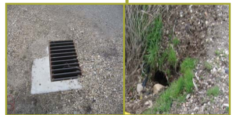
Outfall #9: Victory Rd. and Robinson Rd.
