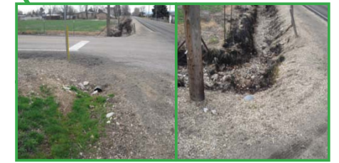
Outfall #10: Orchard Ave. and Pit Ln.
