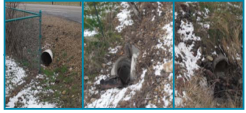
Outfall #6: Lewis Ln. and 12th Ave. Drain
