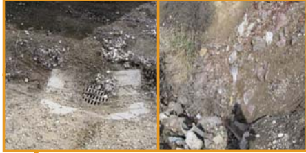
Outfall #2: Portner Rd. and Prairie Ln., Moses Drain
