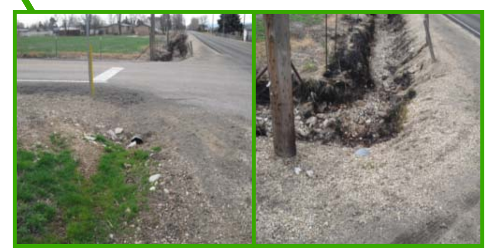
Outfall #10: Orchard Ave. and Pit Ln.
