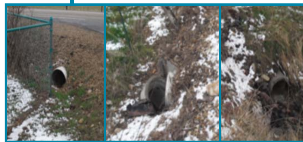
Outfall #6: Lewis Ln. and 12th Ave. Drain
