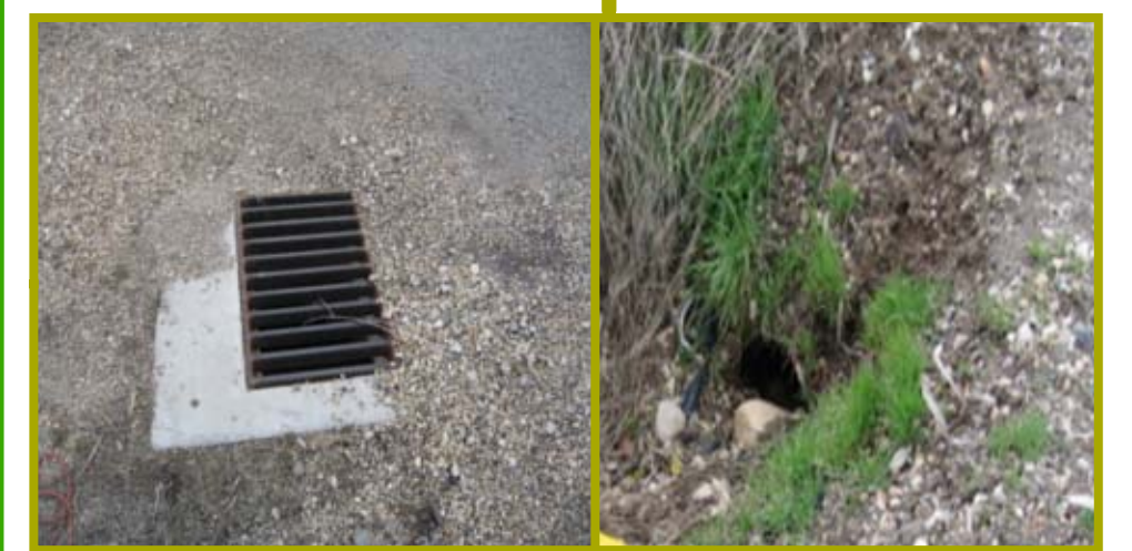
Outfall #9: Victory Rd. and Robinson Rd.
