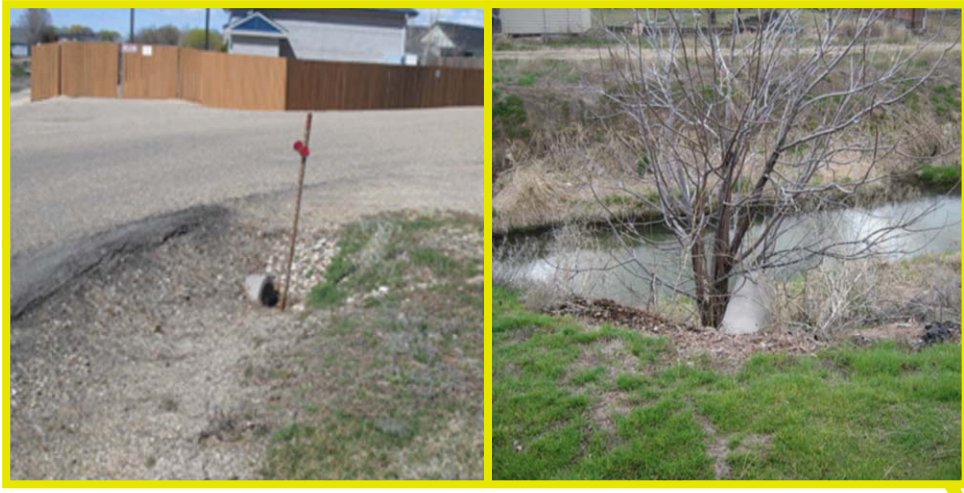
Outfall #1: Oneida St. and Hall Dr., Elijah Drain
