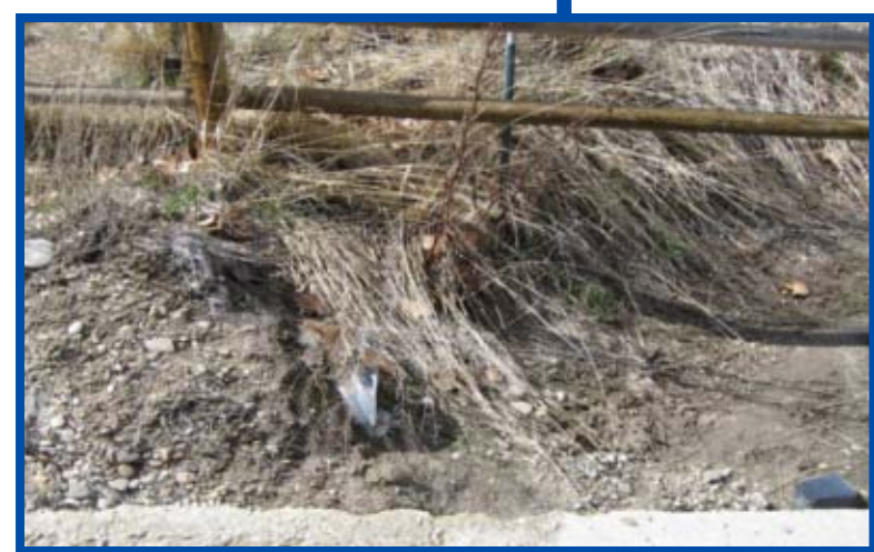
Outfall #8: Sunny Ridge Rd. and North Robinson Lateral
