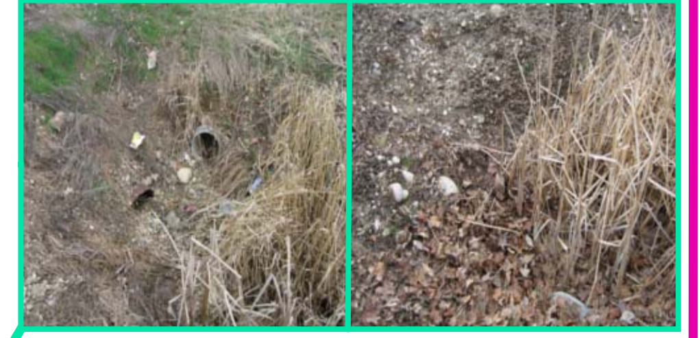
Outfall #5: Star Rd. and Heath Way south side of intersection
