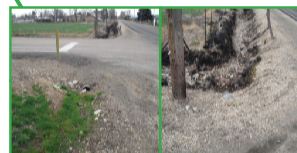
Outfall #10: Orchard Ave. and Pit Ln.
