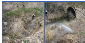
Outfall #12: Star Rd. and Pundam Gulch Drain
