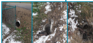
Outfall #6: Lewis Ln. and 12th Ave. Drain
