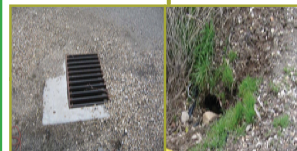
Outfall #9: Victory Rd. and Robinson Rd.
